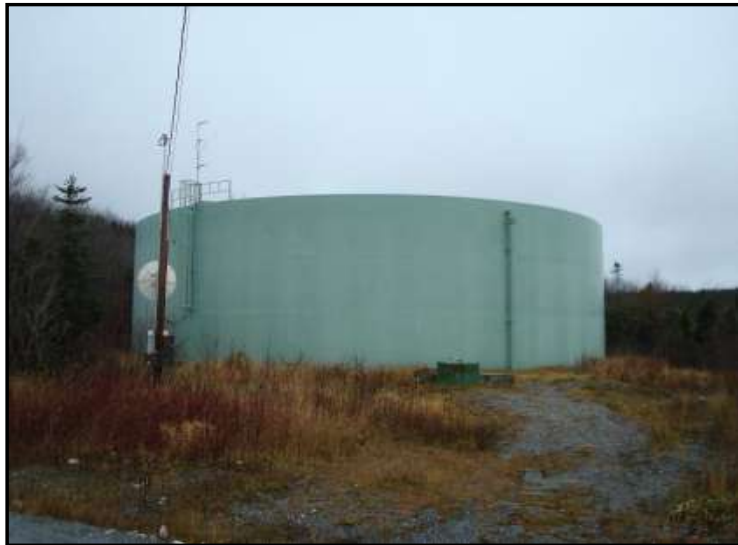
Figure 10. Storage reservoir at Elizabeth Street. (photo by Adam Anderson).
