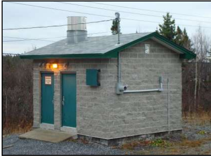
Figure 9. Post-water treatment facility near Lundrigan Drive. (photo by Adam Anderson).
